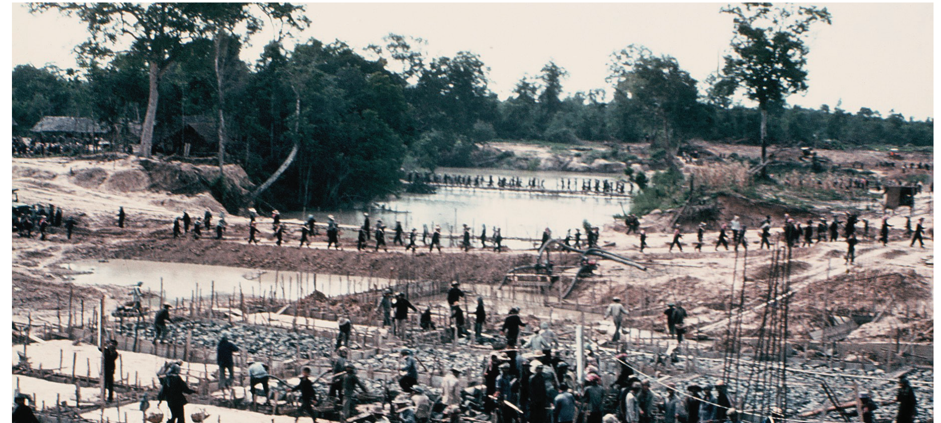
Irrigation dam construction on the road north. Photo by Gunnar Bergstrom
